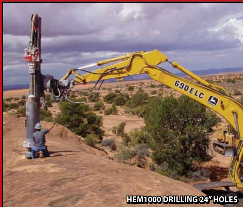
HEM INSTALLING HOLLOW BAR SOIL NAILS
