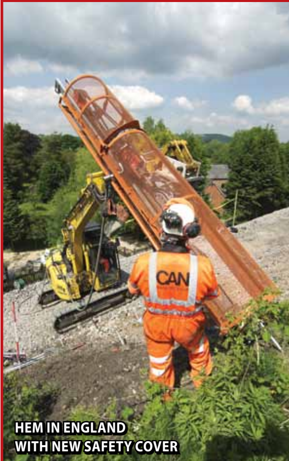
HEM INSTALLING HOLLOW BARS
