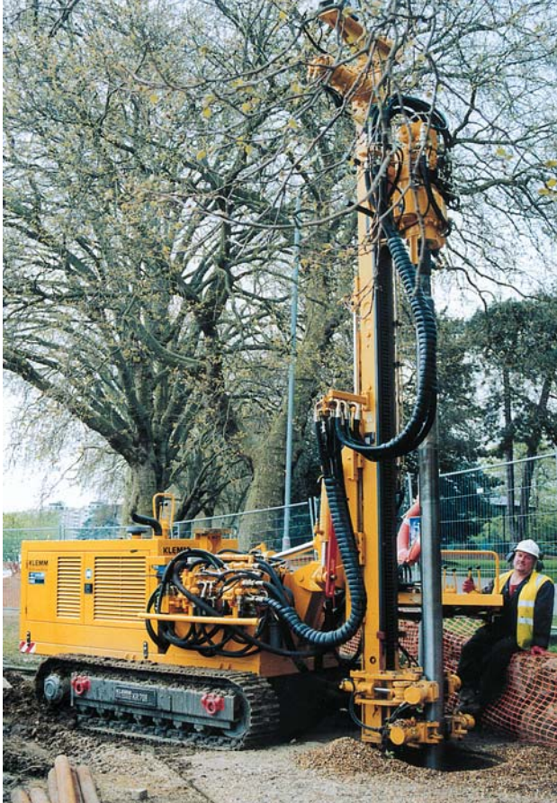
Baustelle England Jobsite England
